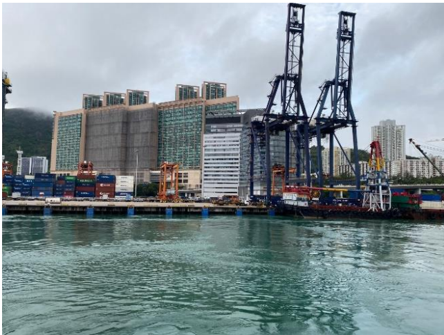
Temporary berth location in HIT at Tsing Yi
